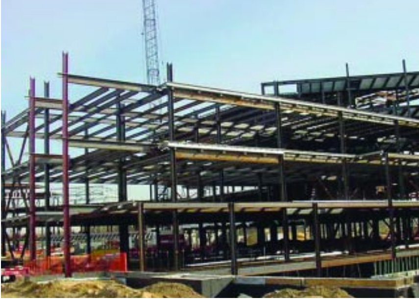
The flexibility of steel framing made it easy to accommodate design changes during construction.
