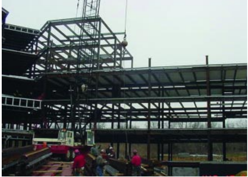
Typical bays consisted of W14 filler beams, W24 girders, and W12 columns.
