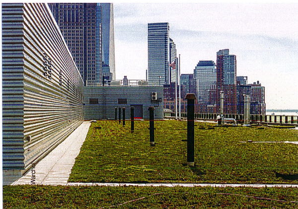
(above) Designed as the building’s fifth façade, the 1.5-acre green roof softens views from neighboring buildings, protects the roof membrane, and enhances storm water retention and thermal performance.
